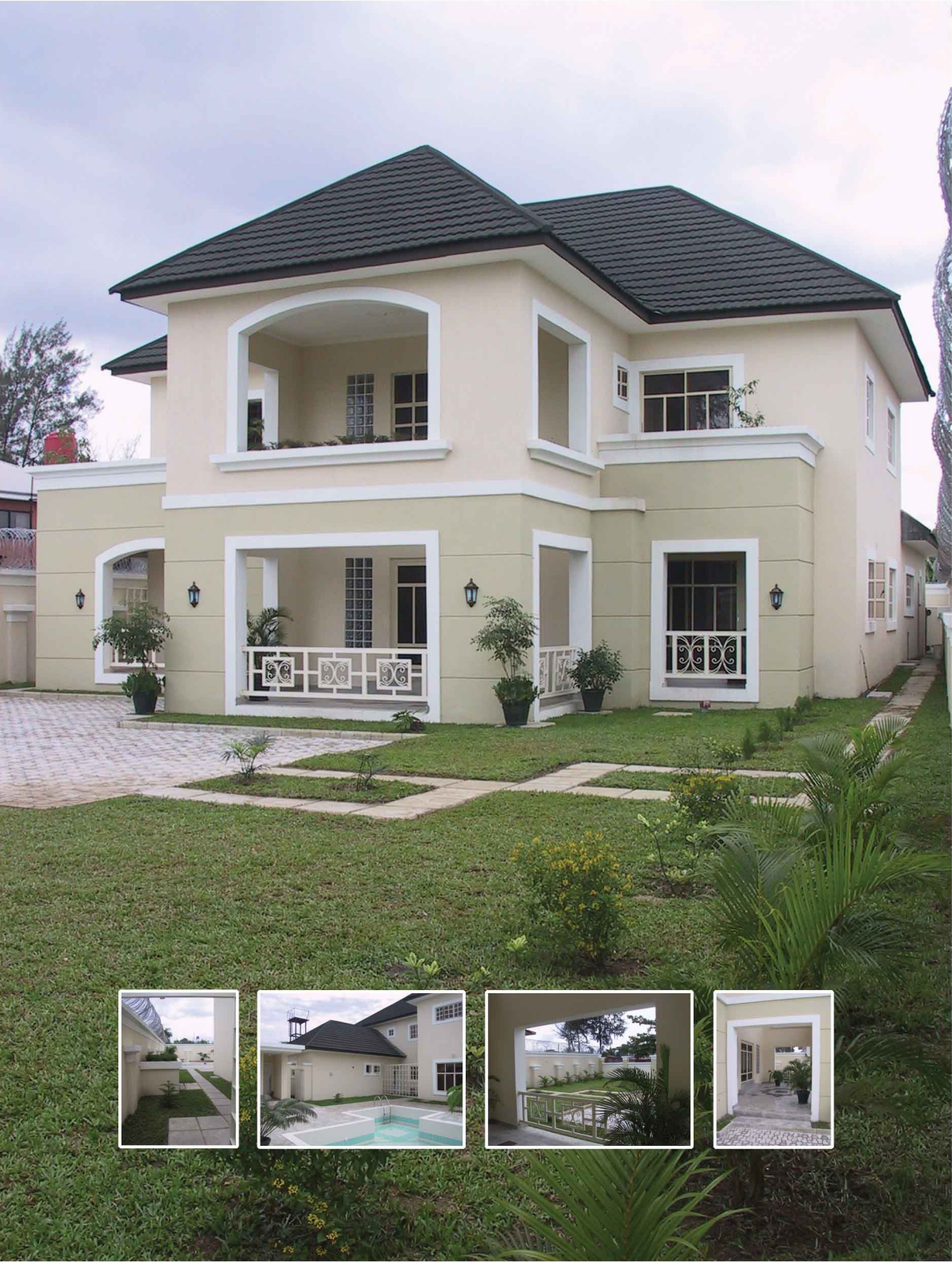
TOP BODO STREET RESIDENCE GRA, PORT HARCOURT.
